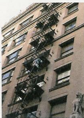
6. a fire escape
