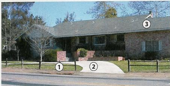
1. a fence 2. a driveway 3. a roof
